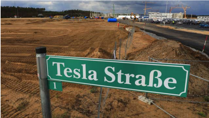
A 'Tesla Street' sign stands near a plot of land at the Tesla Inc. Gigafactory construction site in Gruenheide, Germany, on Wednesday, Sept. 2, 2020.
